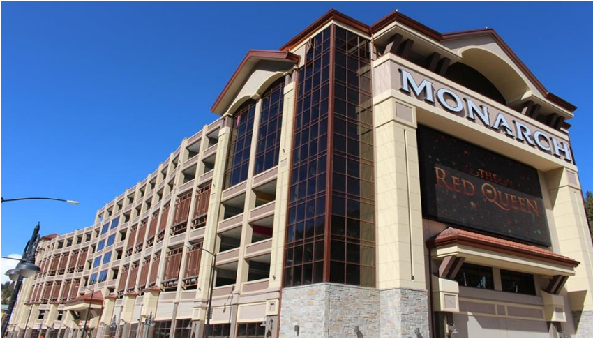
New Parking Structure
