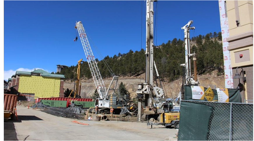
Hotel Tower/Casino Expansion: Current Progress
